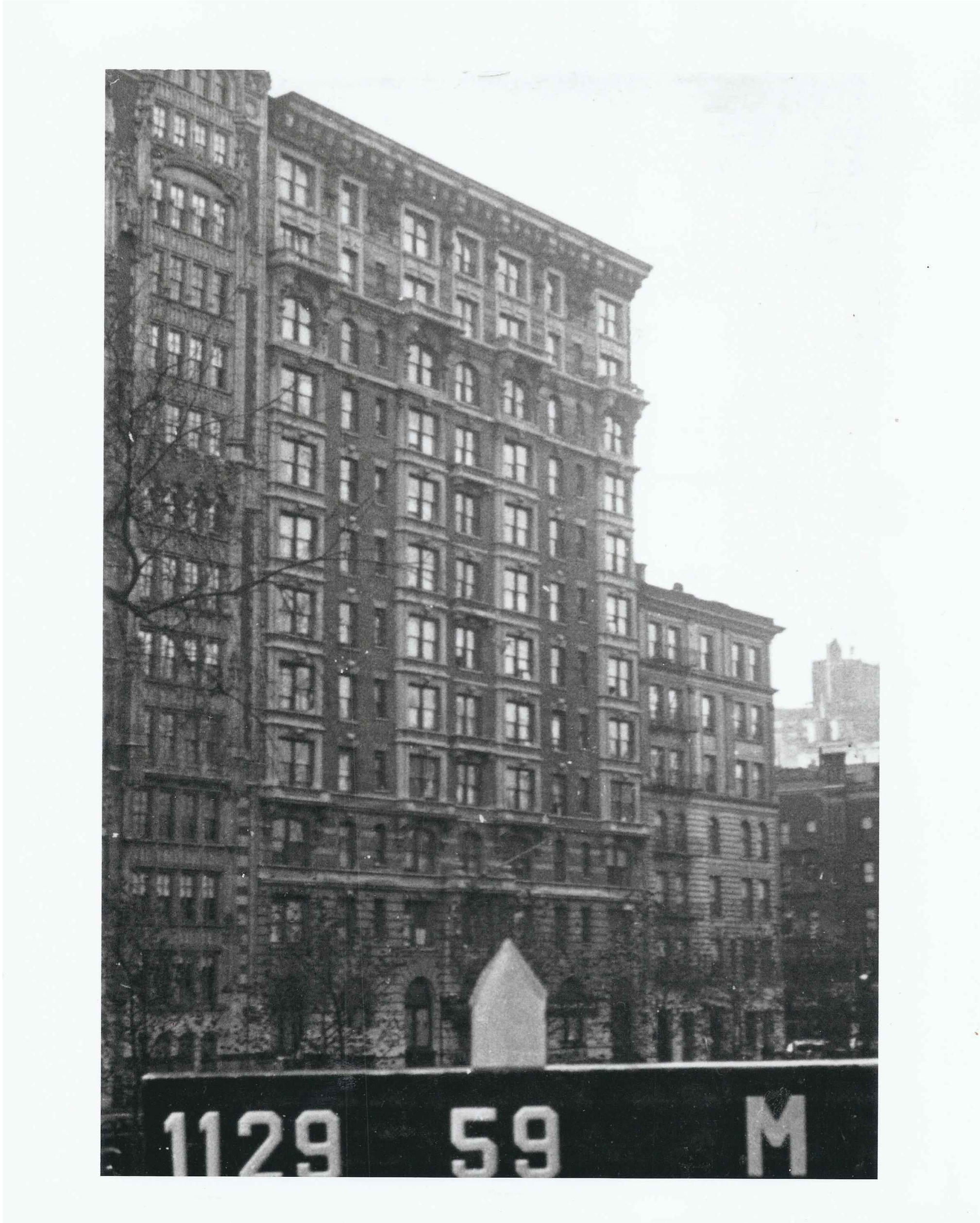
1 ARCHIVAL PHOTOGRAPH LPC-100 1940 TAX PHOTO
